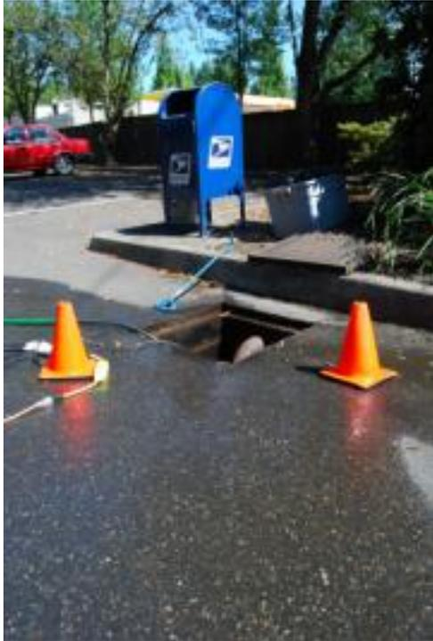
**The goal of this program is to reduce the water pollution risks associated with car wash fundraising events. As part of the program, the City has made available a free sump pump kit that prevents soap and used-washwater from entering the storm sewer system.**
