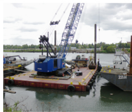
Equipment similar to this crane and barge will appear on the lake in coming months.
