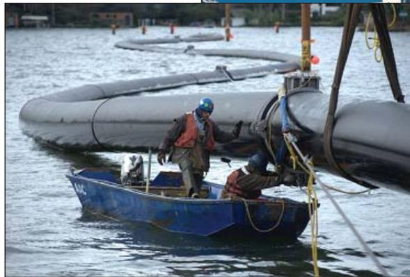
This westward view of Oswego Lake (top) shows construction on the interceptor sewer project during the 24-foot drawdown phase during which pipe-bending operations (left) achieved the pipeline’s sinusoidal shape with the use of internodal cables.
