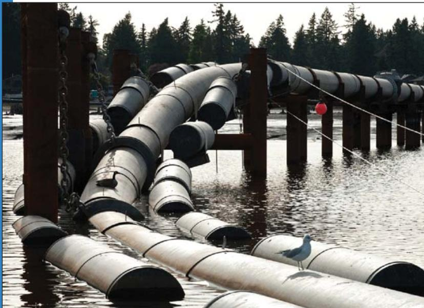
Twin buoyancy pipe modules keep the pipe afloat and transition piles and slings protect the pipe during infrequent major lake drawdowns (left). The artist's rendering (bottom) shows the completed Lake Oswego Interceptor Sewer from below the surface of the lake looking up.
