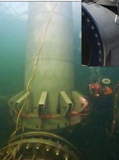
**The Lake Oswego Interceptor Sewer's submerged, buoyant stainless-steel access points provide entry points to the pipeline without affecting boat navigation, and the installation of removable access caissons allows cleaning and inspection equipment to be inserted into for infrequently required maintenance.**
