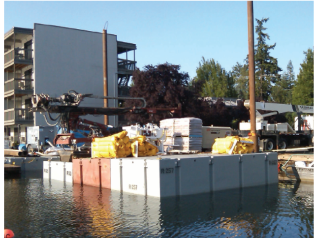
Micropile barge is outfitted near the former US Bank property
