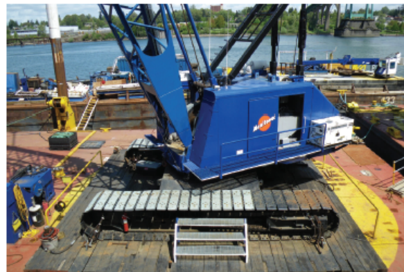
Crane to be staged next to the Lake Corporation marina.
