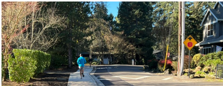
Picture 2: A person using the new Lakewood/Douglas Circle sidewalk.
