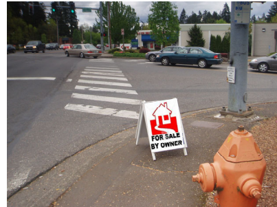
This sign was removed because it obstructs the area between the pedestrian curb ramp and the property line.
