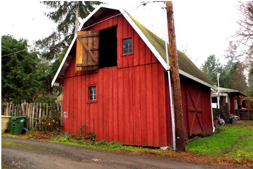
East Façade (Viewing Southwest)
