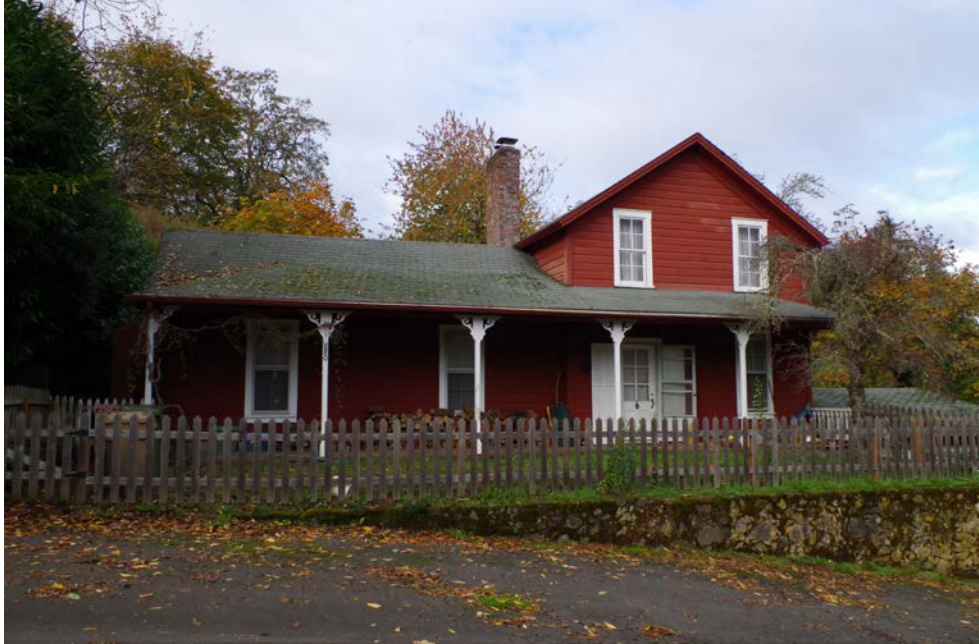
East Façade (Viewing Northwest)
