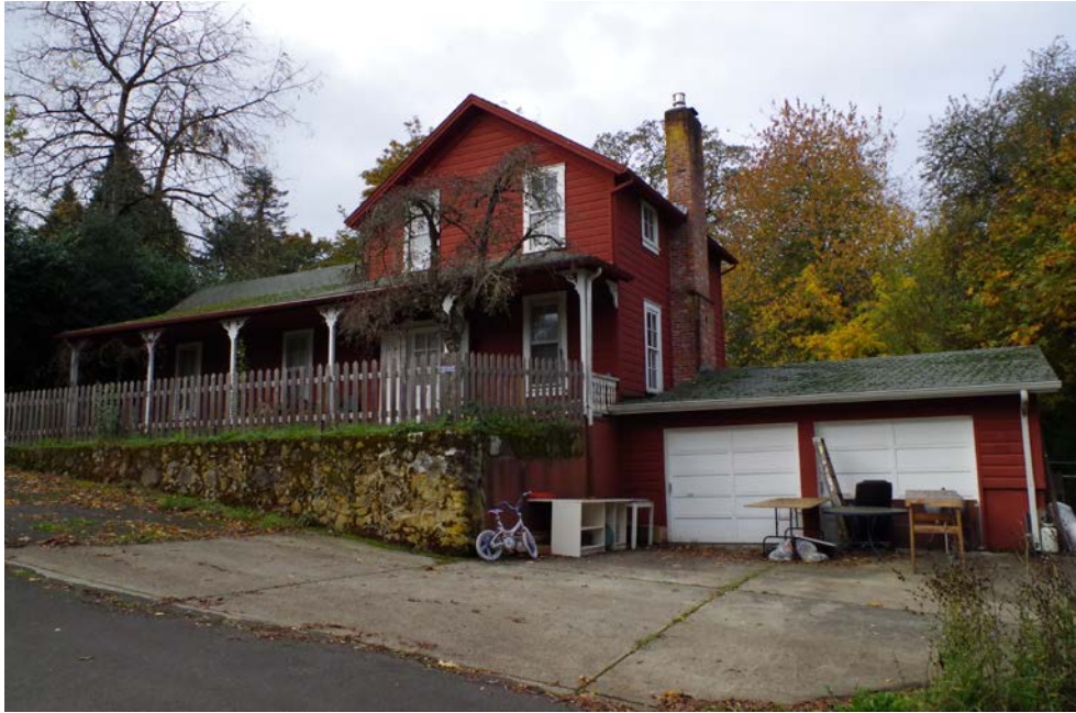
East Façade (Viewing Southwest)
