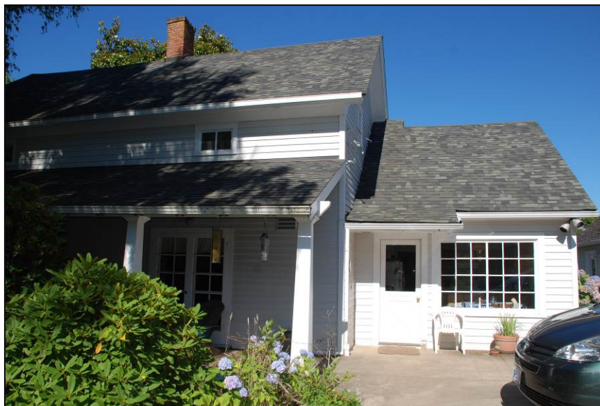
Figure 6: Looking west at the east façade. July 2013
