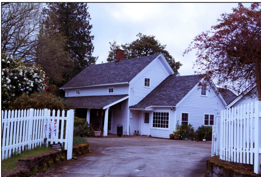
Figure 4: Looking west at the east façade. March 2014
