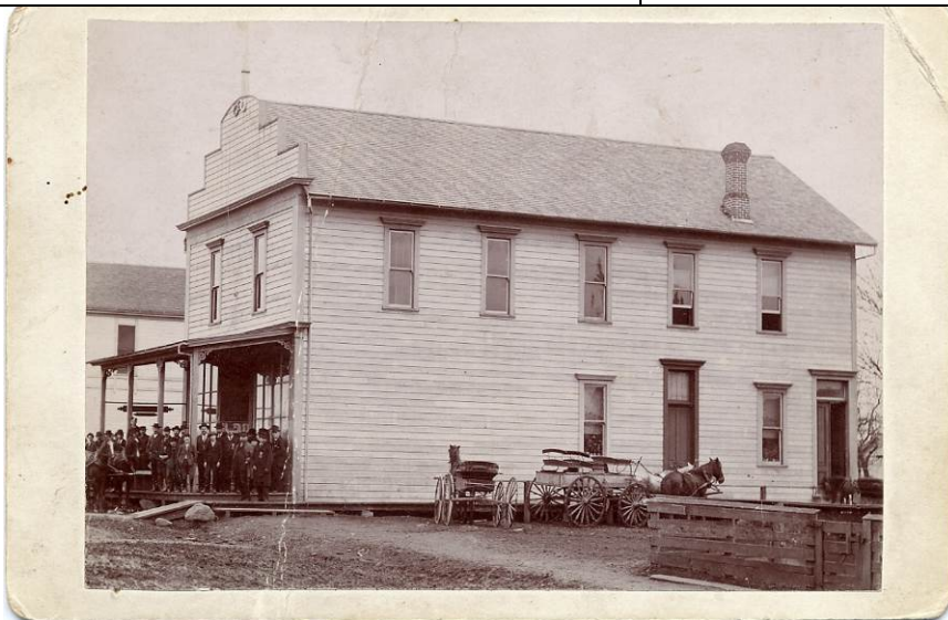
Figure 3: Looking north at the south facade. Date unknown. Photo courtesy of the Lake Oswego Public Library. Photo ID: 3476
