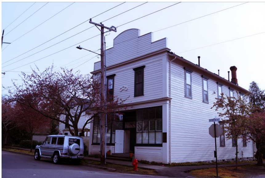
Figure 7: Looking northeast at the south and west façades. 2008.
