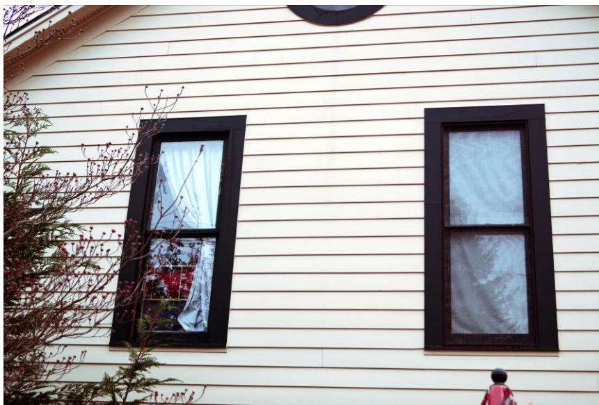
Figure 9: compatible windows on addition. Looking east at the west façade. March 2014.
