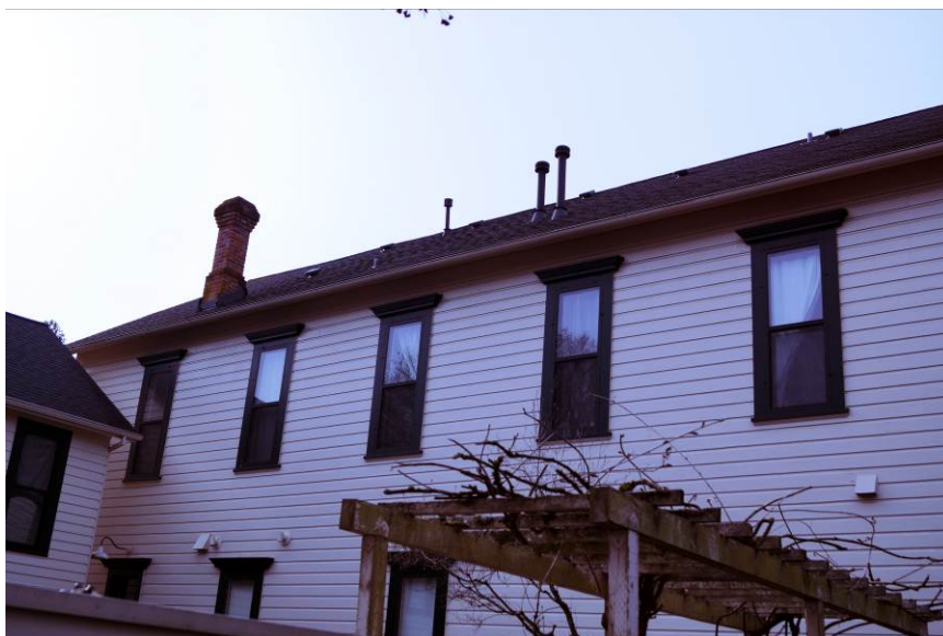
Figure 10: Looking southeast at the north façade. March 2014.
