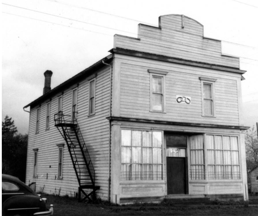
Figure 4: Looking southeast at the west and north façades. 1959. Photo courtesy of the Lake Oswego Public Library. Photo ID:5662
