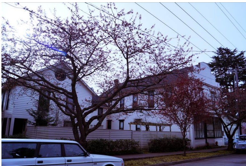
Figure 8: Looking southeast at the west and north façades. March 2014.
