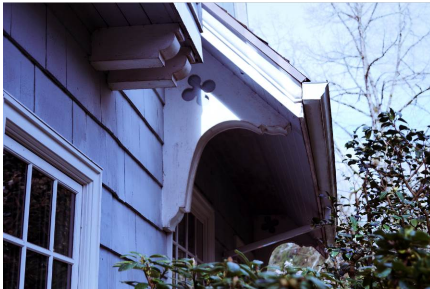
Figure 8: Bracket detail on North facade. March 2014.
