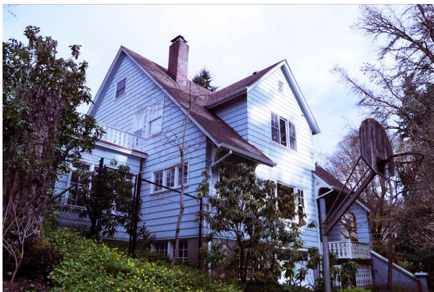
Figure 6: Looking northeast at the south and west façades. March 2014.
