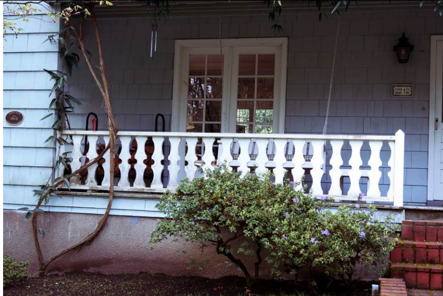
Figure 7: Detail of the porch rails on the north (primary) facade. March 2014
