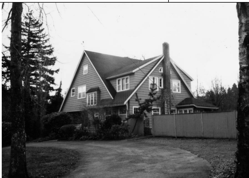
Figure 3: Looking south at the north and east façades. ca. 1989. Photo courtesy of the Lake Oswego Public Library. Photo ID: HRAB118
