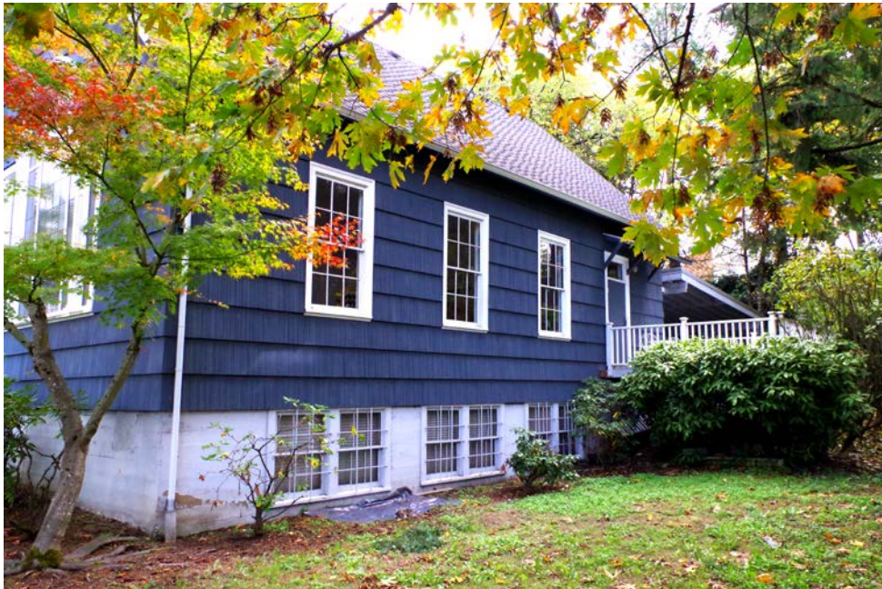
West Façade (Viewing Southeast)
