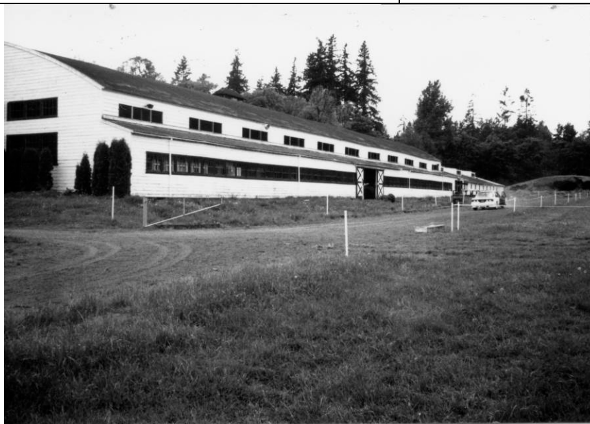
Figure 3: Looking southwest at the north façade. No date. Photo courtesy of the Lake Oswego Public Library. Photo ID: HRAB159
