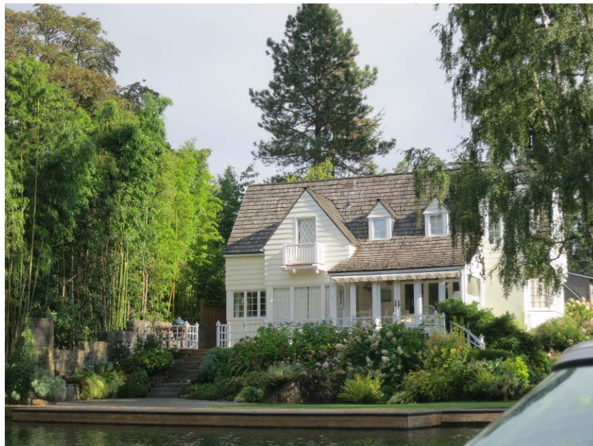
Figure 4: Looking north at the south façade. Courtesy of the Lake Oswego Library: Photograph ID 6412. 2013.
