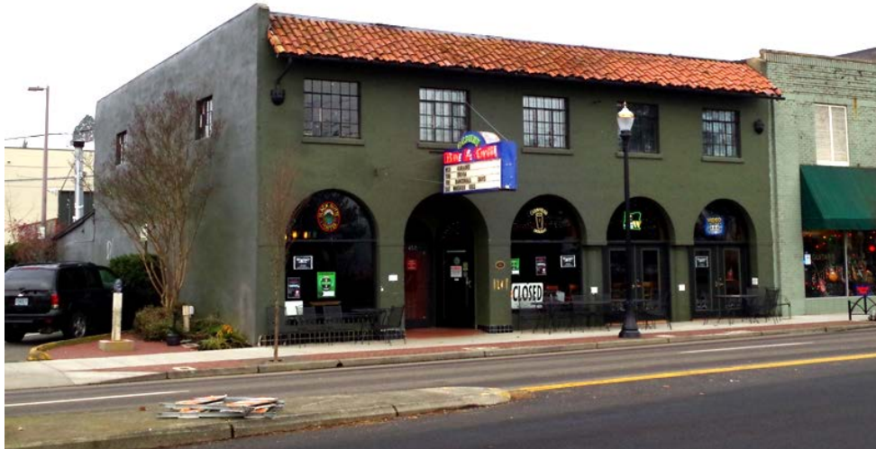
East Façade (Viewing Northwest)
