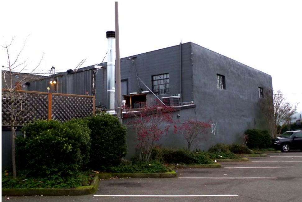
South Façade (Viewing Northeast)
