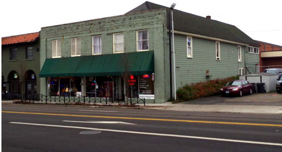
East Façade (Viewing Southwest)
