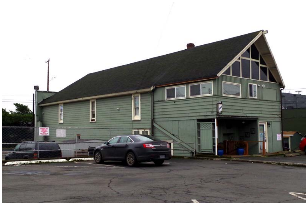
North Façade (Viewing Southeast)
