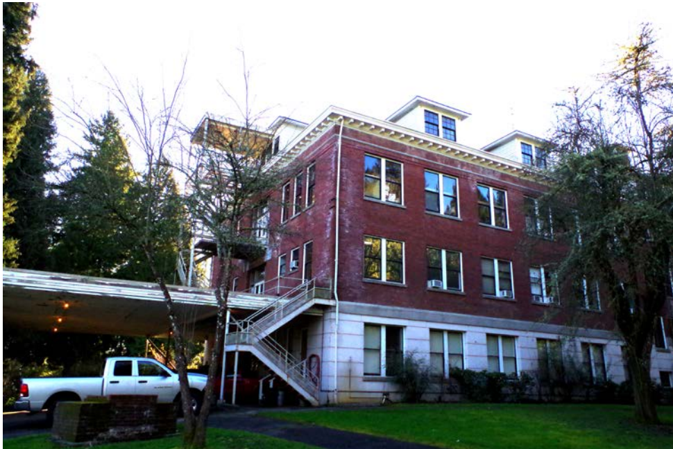
North Façade (Viewing Southwest)
