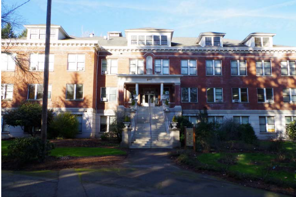
South Façade (Viewing North)
