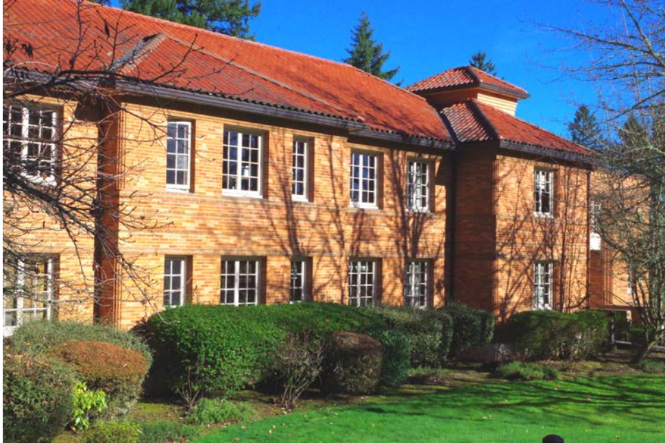
South Façade (Viewing Northeast)
