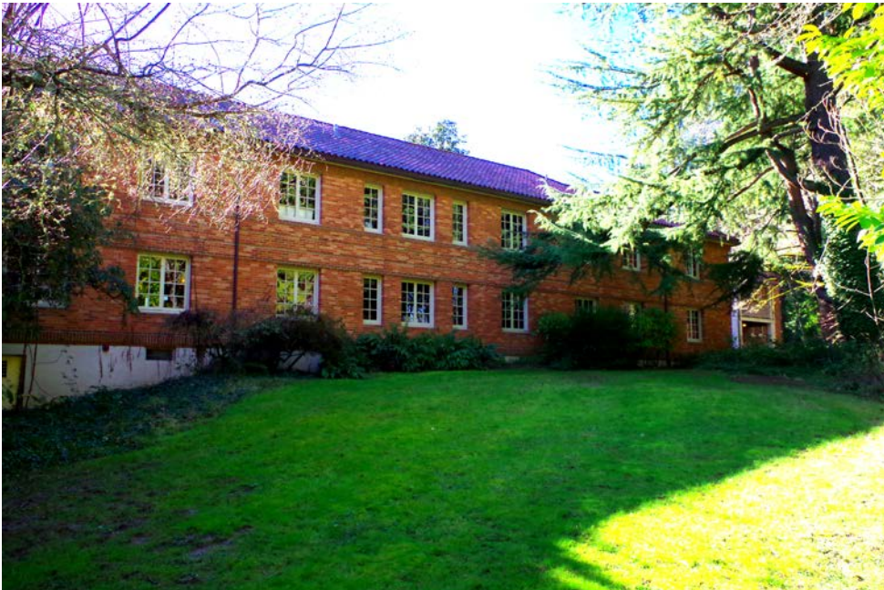
North Façade (Viewing Southwest)
