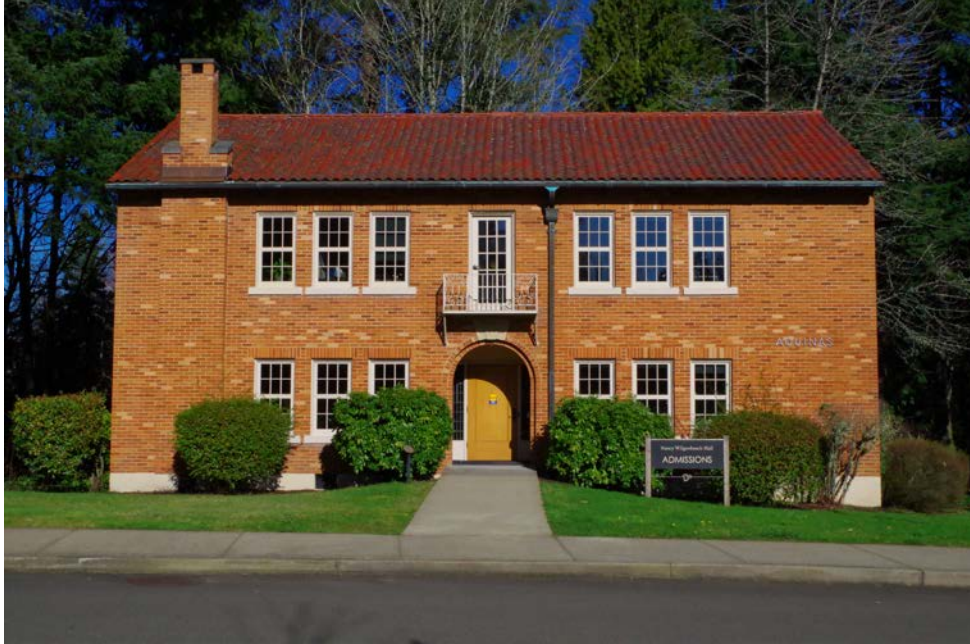
South Façade (Viewing North)
