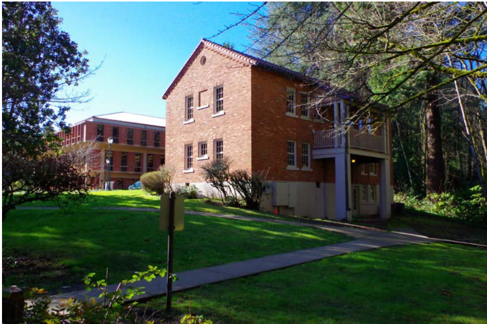
East Façade (Viewing Southwest)
