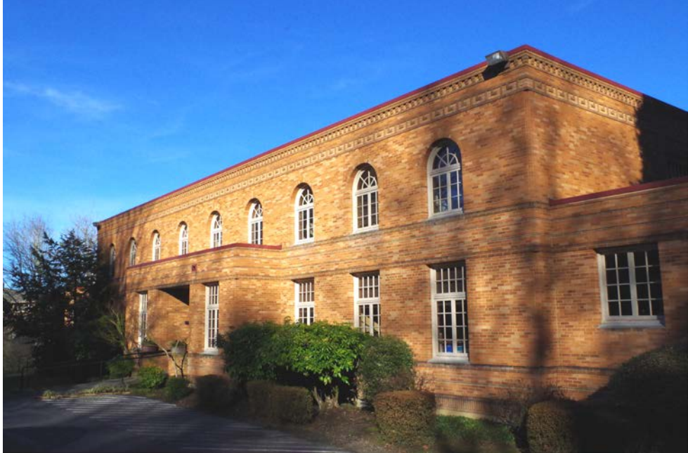
West Façade (Viewing Northeast)
