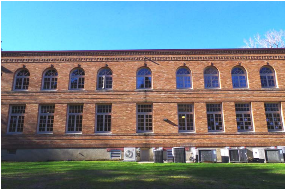
East Façade (Viewing West)
