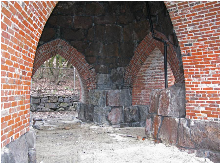
Figure 12. Blast House. 2010. Photo by Susanna Kuo
