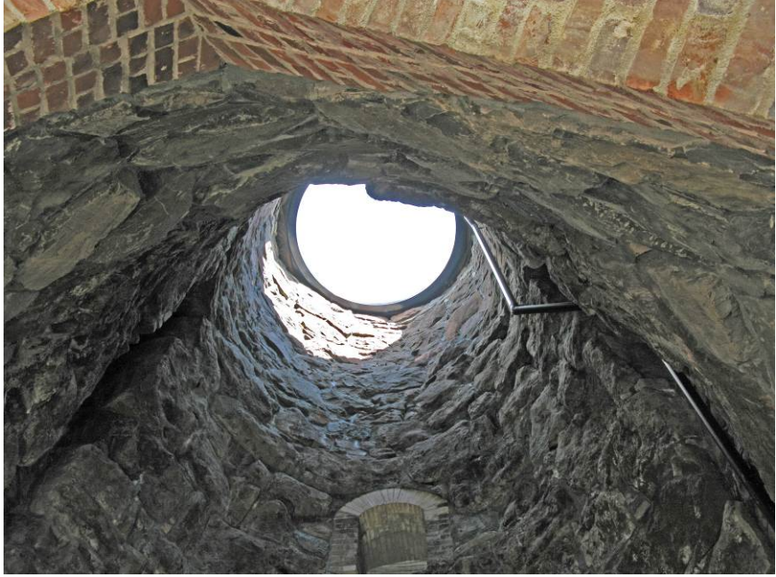
Figure 13. Furnace, interior, looking up, George Rodgers Park. 2010 Photo by Susanna Kuo
