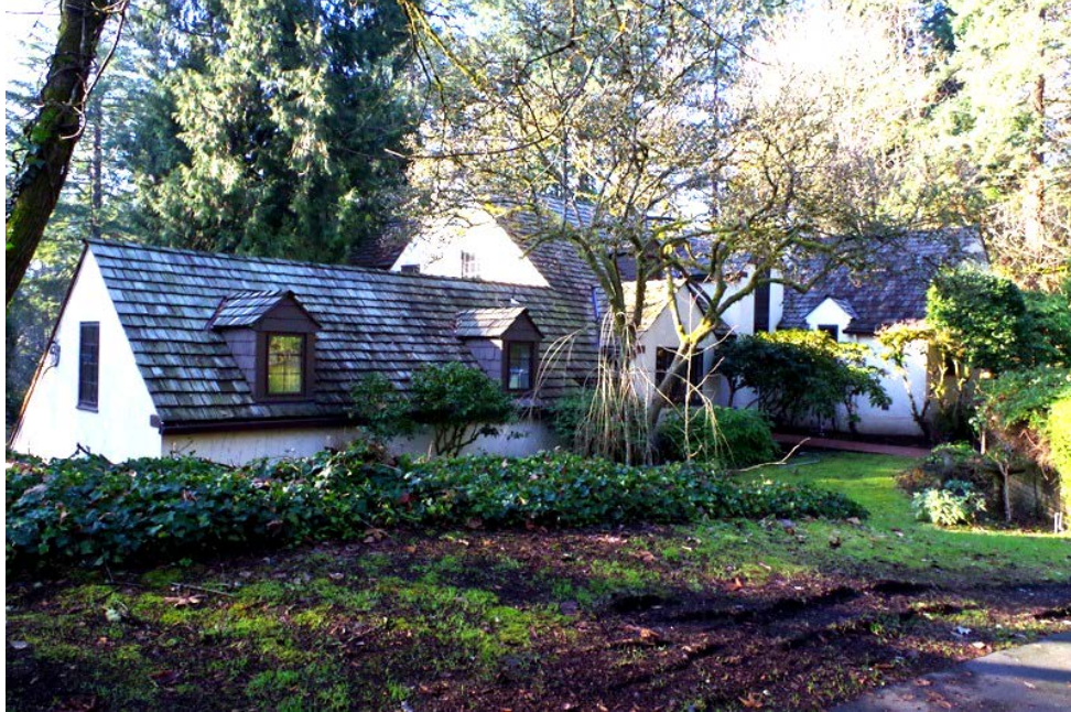
North Façade (Viewing Southwest)
