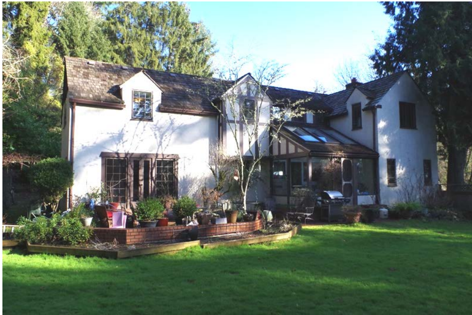
South Façade (Viewing Northeast)
