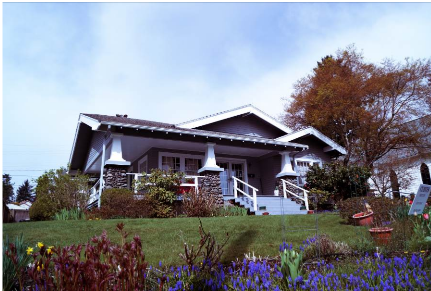
Figure 7: Looking northwest at the east and south façades. March 2014.
