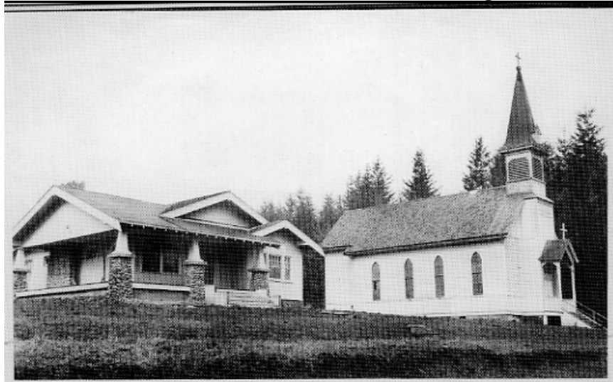
Figure 4: Looking northwest at the south and east façades. Date unknown. On file at the Catholic Press, Portland, Oregon.
