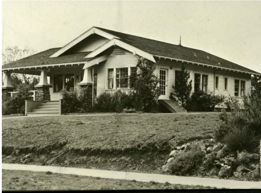
Figure 3: Looking southwest at the north and east façades. Date unknown. On file at the Catholic Press, Portland, Oregon.
