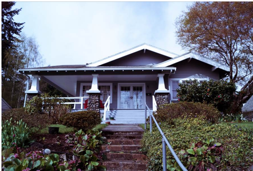
Figure 8: Looking west at the east façade. March 2014.
