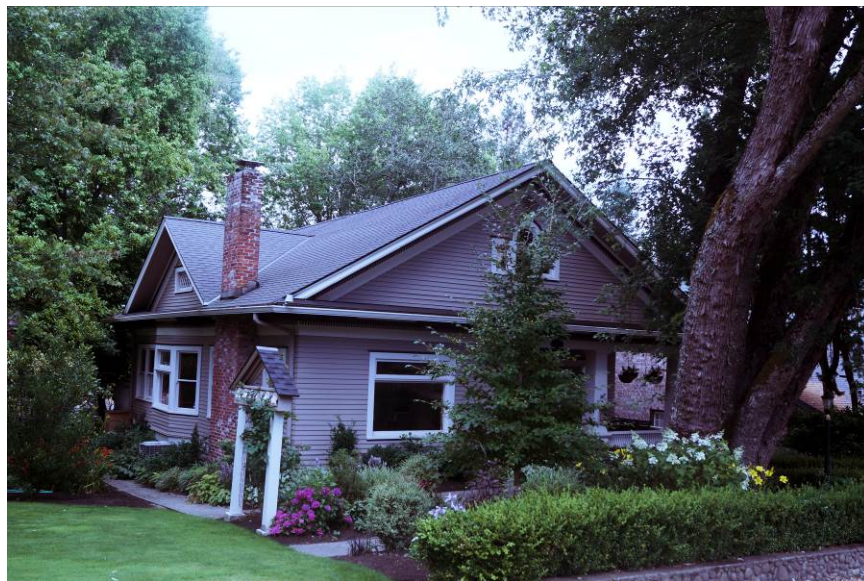
Figure 4. Looking southeast at the north and west façades. March 2014.
