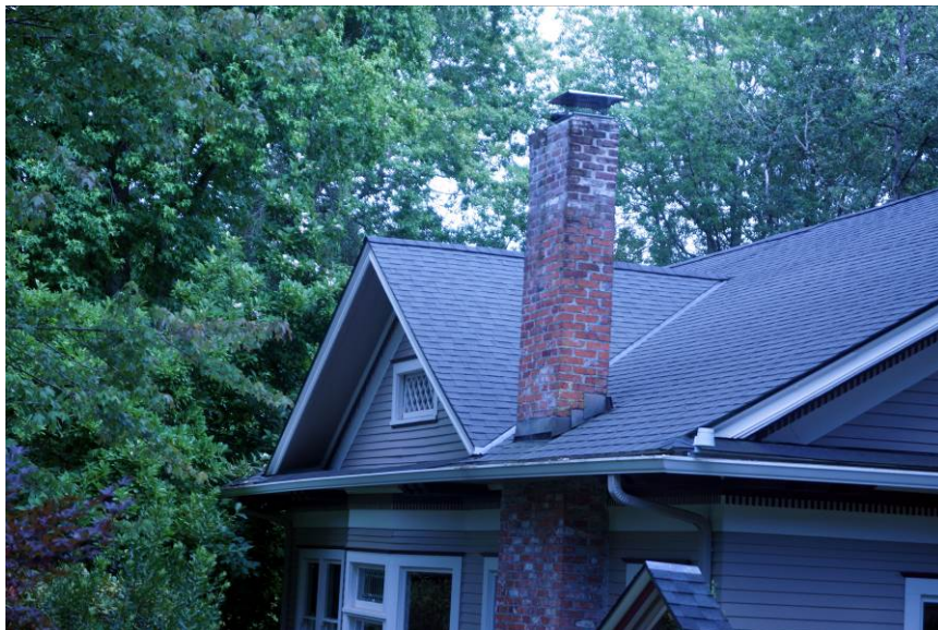
Figure 6. Detail of chimney and wall gable with lattice window. March 2014.
