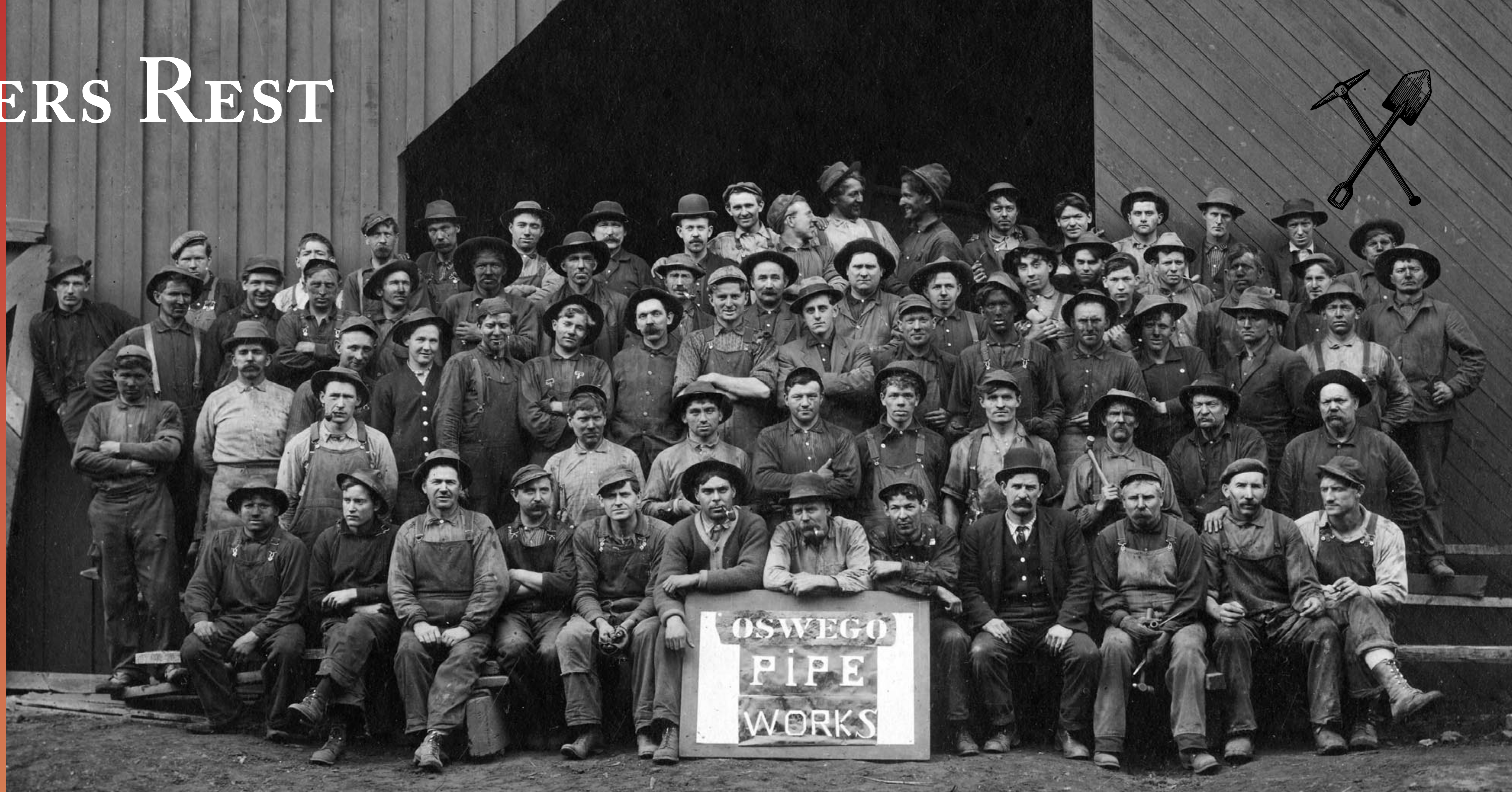
Oswego Pipe Foundry crew, c. 1915. Courtesy of the Lake Oswego Public Library. Workers buried in the Oswego Pioneer Cemetery.
