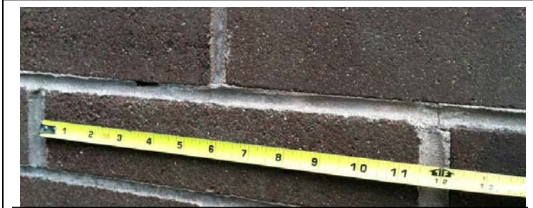
Typical 2.5 x 11-inch brick siding on the Taylor-Made Labels facility.
