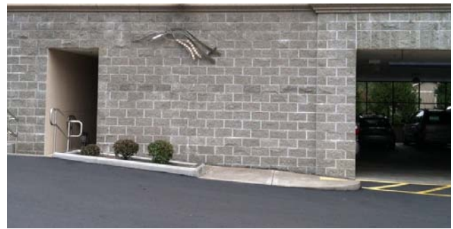
CMU block base on the Crossing building.
