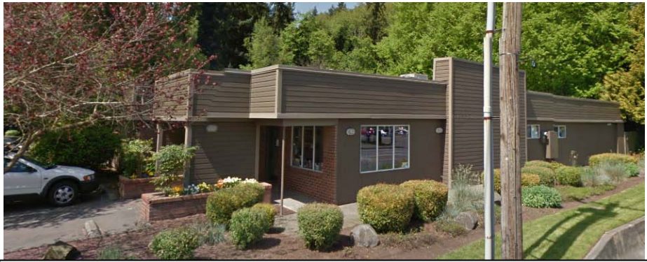
Lake Grove Vet Clinic at 17131 Boones Ferry Road. Exterior cladding is vertical and horizontal siding with some brick.
