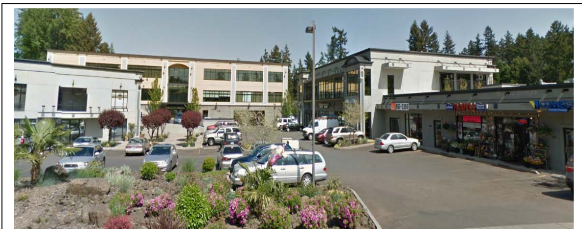
The Crossing, a mixed use office and commercial center. Exterior cladding is stucco with some CMU block at the base of the office building.
