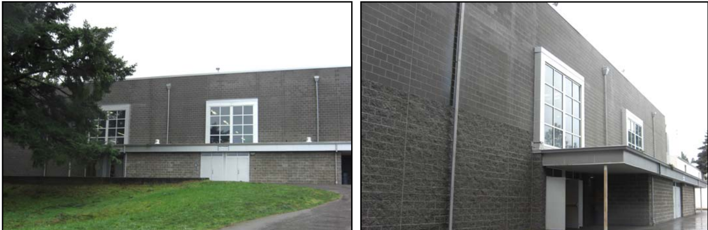
Smooth and split faced CMU in charcoal, metal panels and substantial trim on gymnasium
